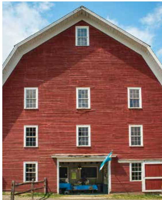
Previous pages: Ransom Conant outside the 1915 barn at his family’s dairy farm in Richmond, Vermont. Opposite: Preservation contractor Eliot Lothrop inside Conant’s barn. This page, top to bottom: Conant, his wife, Alison, and their daughter, CC, with a few of their Holstein cows; The building’s traditional gambrel roof and six-over-six windows.
